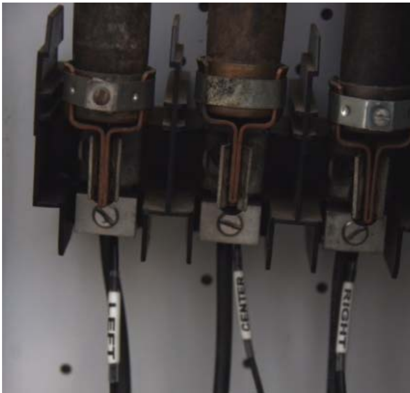
Figure 7 – Voltage Measurement Connections
