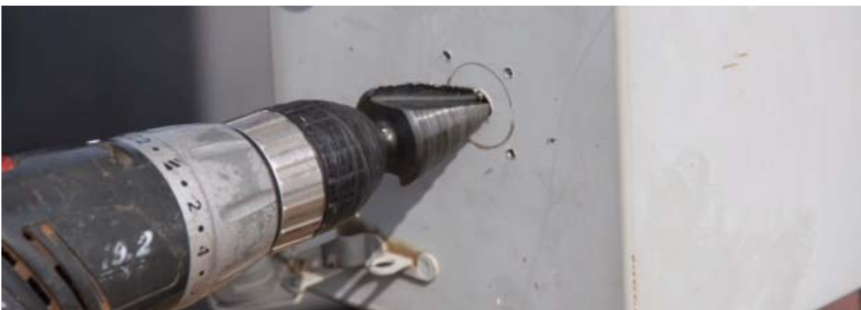
Figure 4 – Step Drill Center Hole
